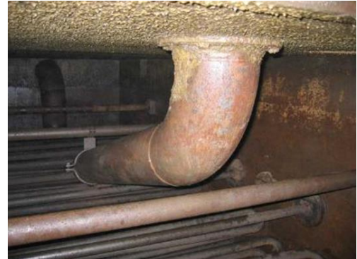
Smeerolie tank (25 m 3 ) na reinigen
