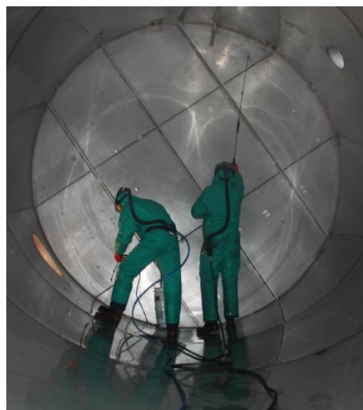
Spray pickling of a stainless steel tank
