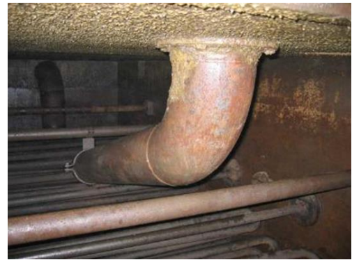
Lub oil tank (25 m 3 ) after cleaning
