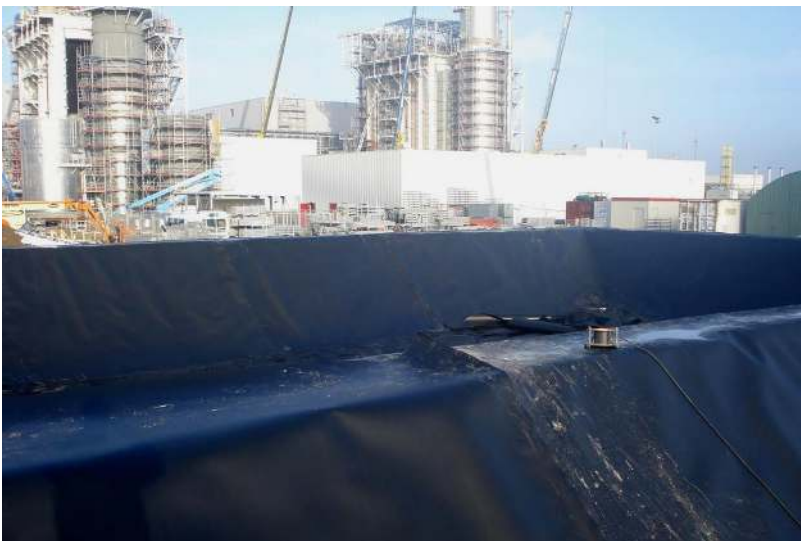
Foil with in the background the HRSGs that have now been cleaned that are still partly being built
