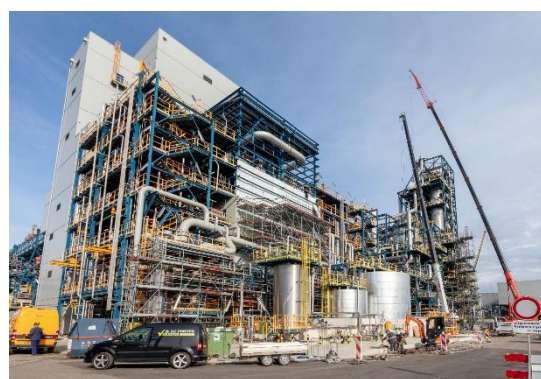
Pre-commission cleaning on the basis of EDTA
